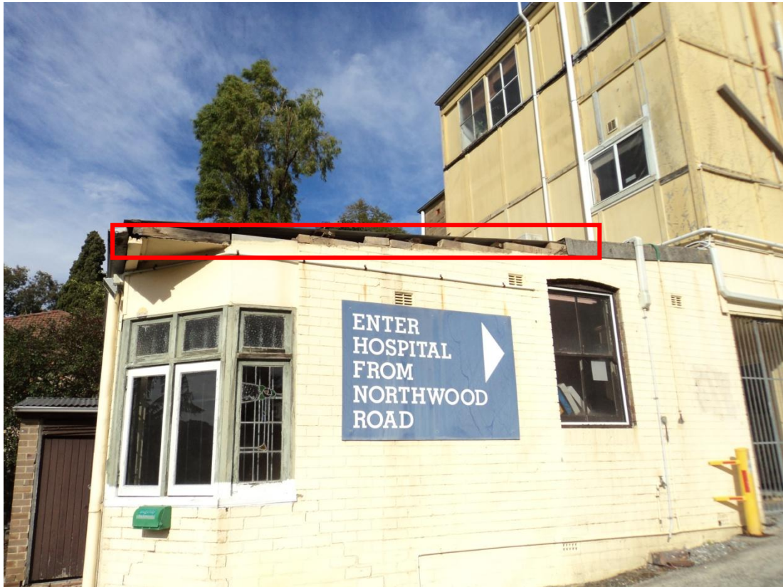
Photograph 3.10 Crevices in roofing (outlined in red) suitable for microbats
